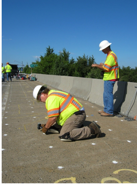
Figure 2-13 Bridge deck sounding with a hammer.
