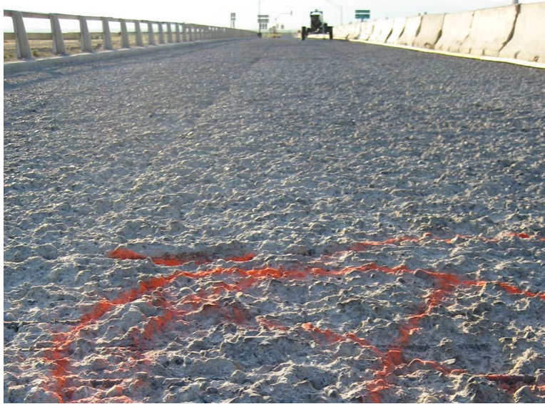
Figure 2-41 Surface prepared for concrete overlay (Nolan 2008).
