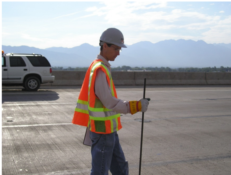
Figure 2-14 Bridge deck sounding with an iron bar.
