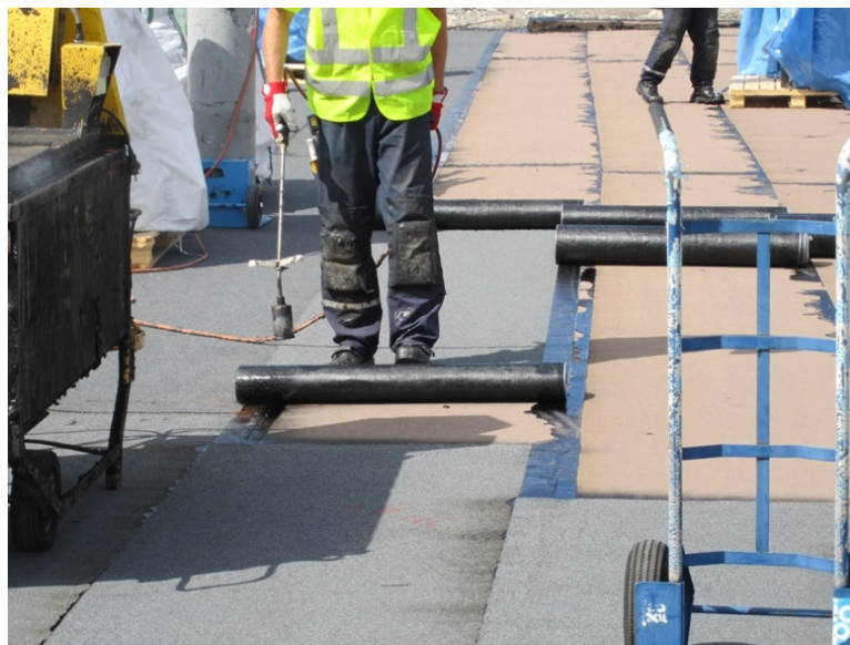
Figure 2-39 Preformed membrane application process.
