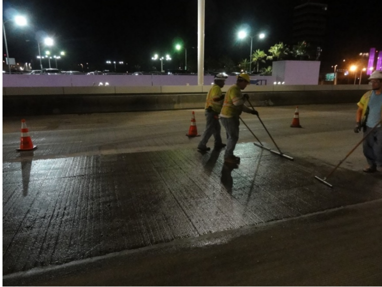
Figure 2-36 Methacrylate sealant application process.
