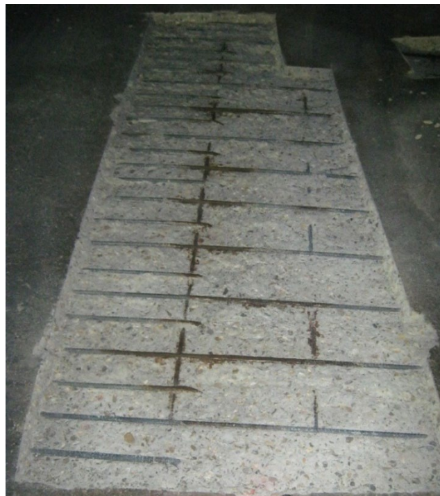
Figure 2-43 Cover concrete removal.
