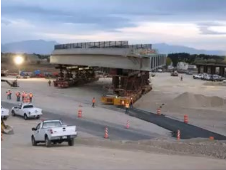
Figure 2-49 Movement of a bridge using mobile transporters.
