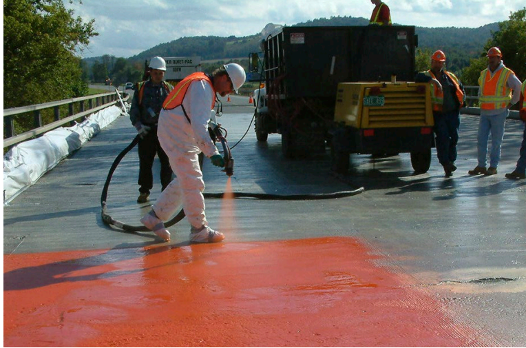
Figure 2-40 Spray-applied membrane application process (Bridge Preservation 2016).
