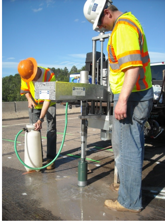
Figure 2-4 Coring of a concrete bridge deck.
