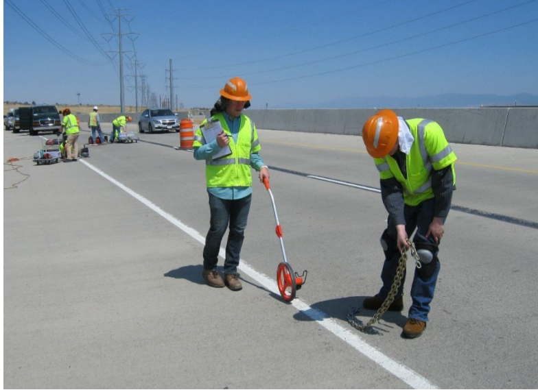
Figure 2-1 Chain dragging of a concrete bridge deck.
