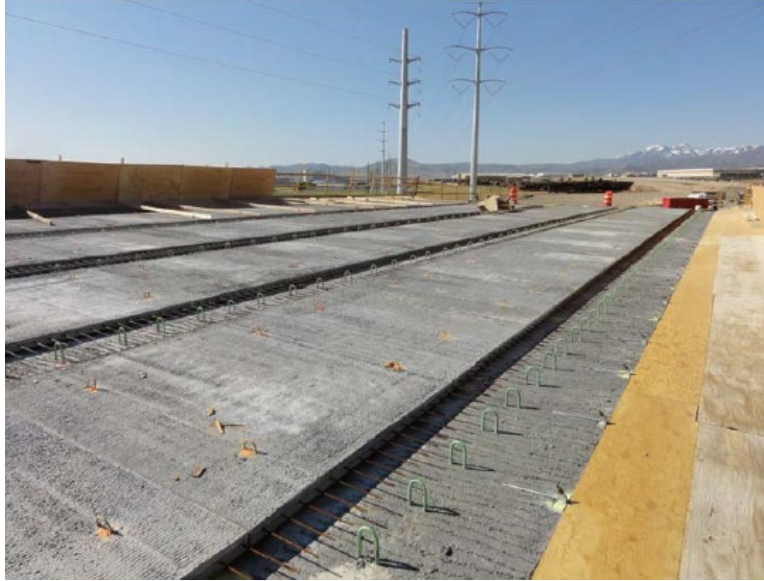
Figure 2-46 Precast half-deck panels.
