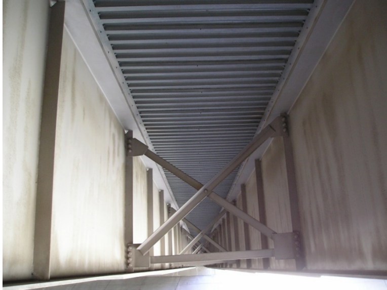
Figure 2-45 Bottom view of SIPMF (Guthrie et al. 2006).
