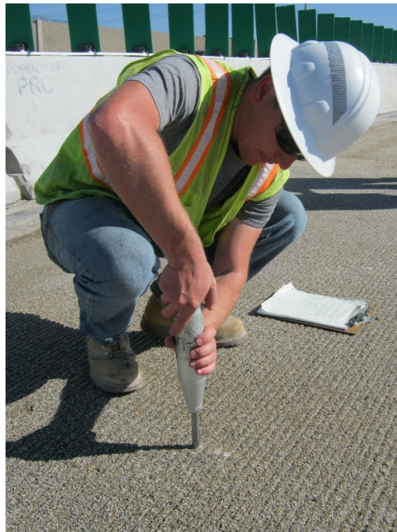
Figure 2-26 Schmidt rebound hammer testing.
